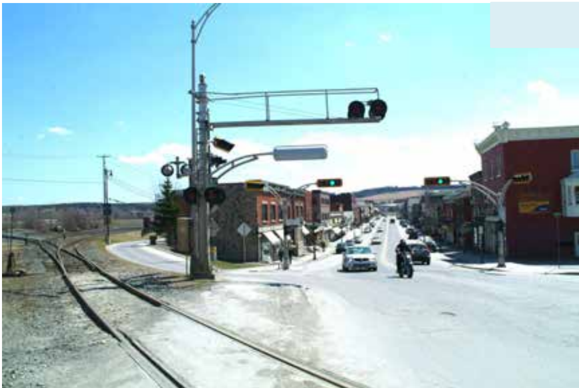
Figure 8: Switch and curve where the derailment likely occurred
