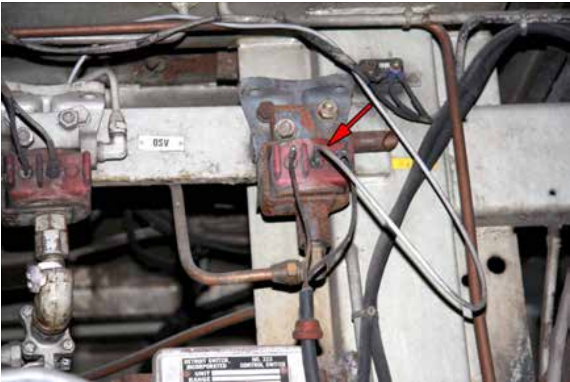
Figure 7: “Brake Test” connection for locomotive 5023
