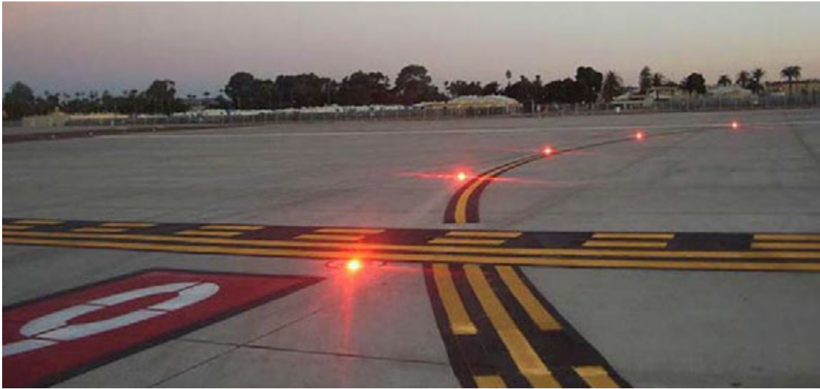
Figure 22. Example of lit runway entrance lights (Source: U.S. Federal Aviation Administration, "Runway Status Lights Photo Gallery," at https://www.faa.gov/air_traffic/technology/rwsl/gallery [last accessed 31 December 2018])
