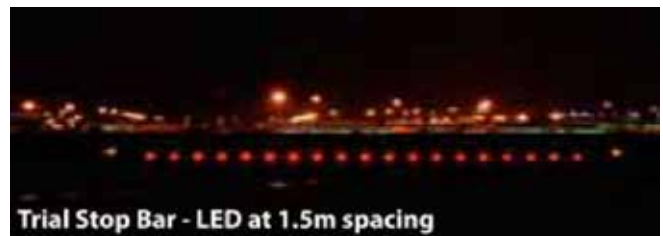
Figure 10. Reduced stop-bar light spacing with LED lights (Source: EUROCONTROL, Hindsight 19 [2014], p. 18)
