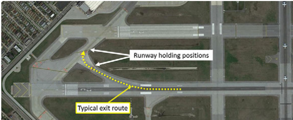
Figure 20. Chicago Midway International Airport (KMDW), Illinois, U.S. has the only identified example, other than CYYZ, of a runway holding position located after a significant turn on a rapid exit taxiway in North America. (Source: Google Earth, with TSB annotations)
