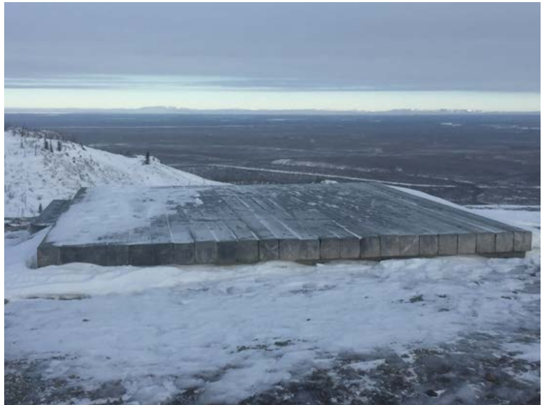
Figure 1. Helipad on Bear Rock (Source: Great Slave Helicopters Ltd.)
