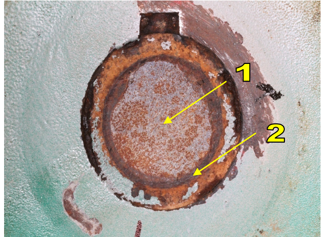
Photo 4. A close-up of the outboard end of the fractured west idler wheel axle, after cleaning 1. Overstress failure (90%) 2. Fatigue cracking around the periphery at the change of cross section. The corrosion indicates that the cracks had been present for some time.
