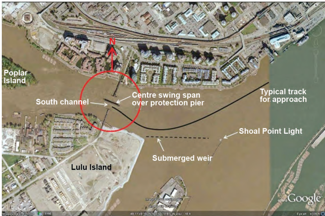
Photo 4. Queensborough Railway Bridge approach
