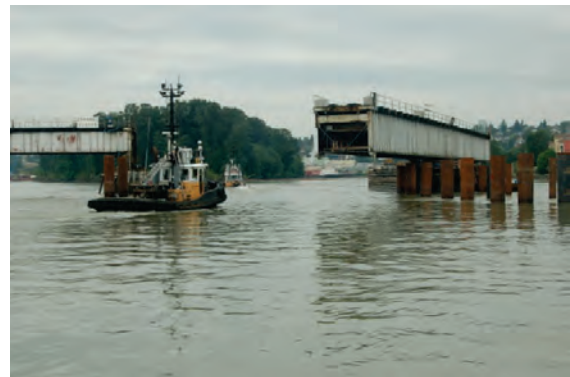
Photo 3. Queensborough Railway Bridge
