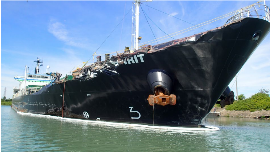
Figure 9. Damage to the forward starboard section of the Florence Spirit 's hull (Source: TSB)
