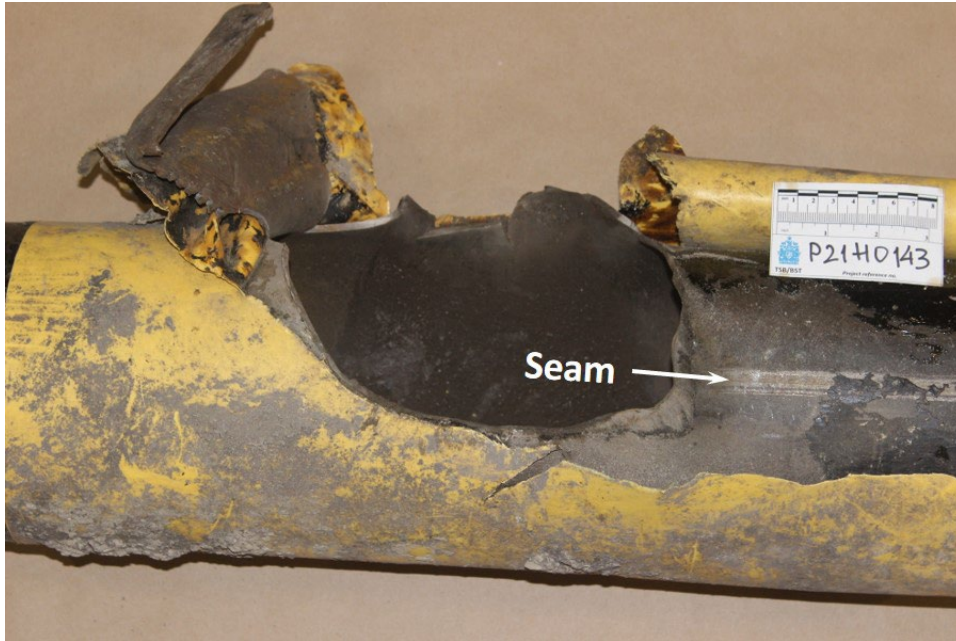
Figure 8. Segment of pipe where damage occurred (Source: TSB)
