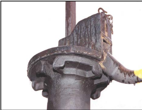
Figure 17 - Top photographs show switch points open 3/16 inch yet a green CTC signal is displayed to a train crew. Bottom photographs show an unlocked and partially raised switch handle, yet a green switch target.
