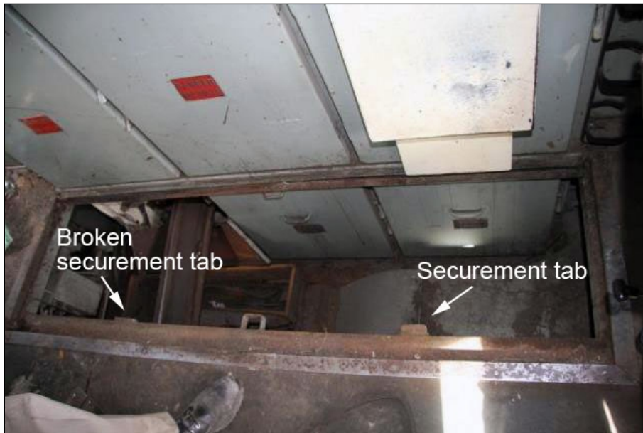
Photo 2. Floor panel cavity
