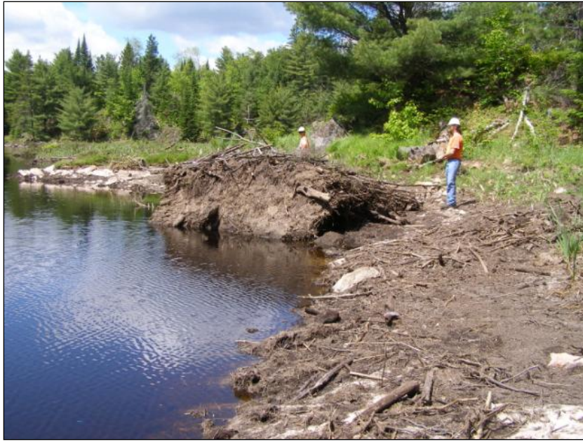
Photo 4. Displaced portion of beaver dam
