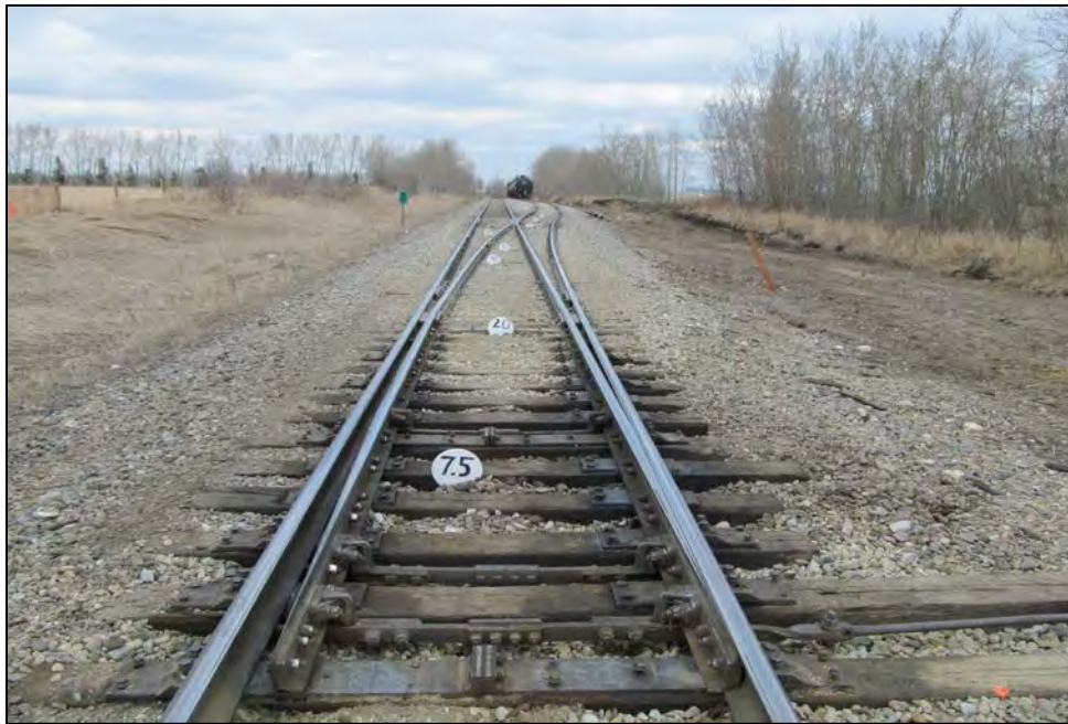
Photo 5. Looking north, south siding turnout at Campaign
