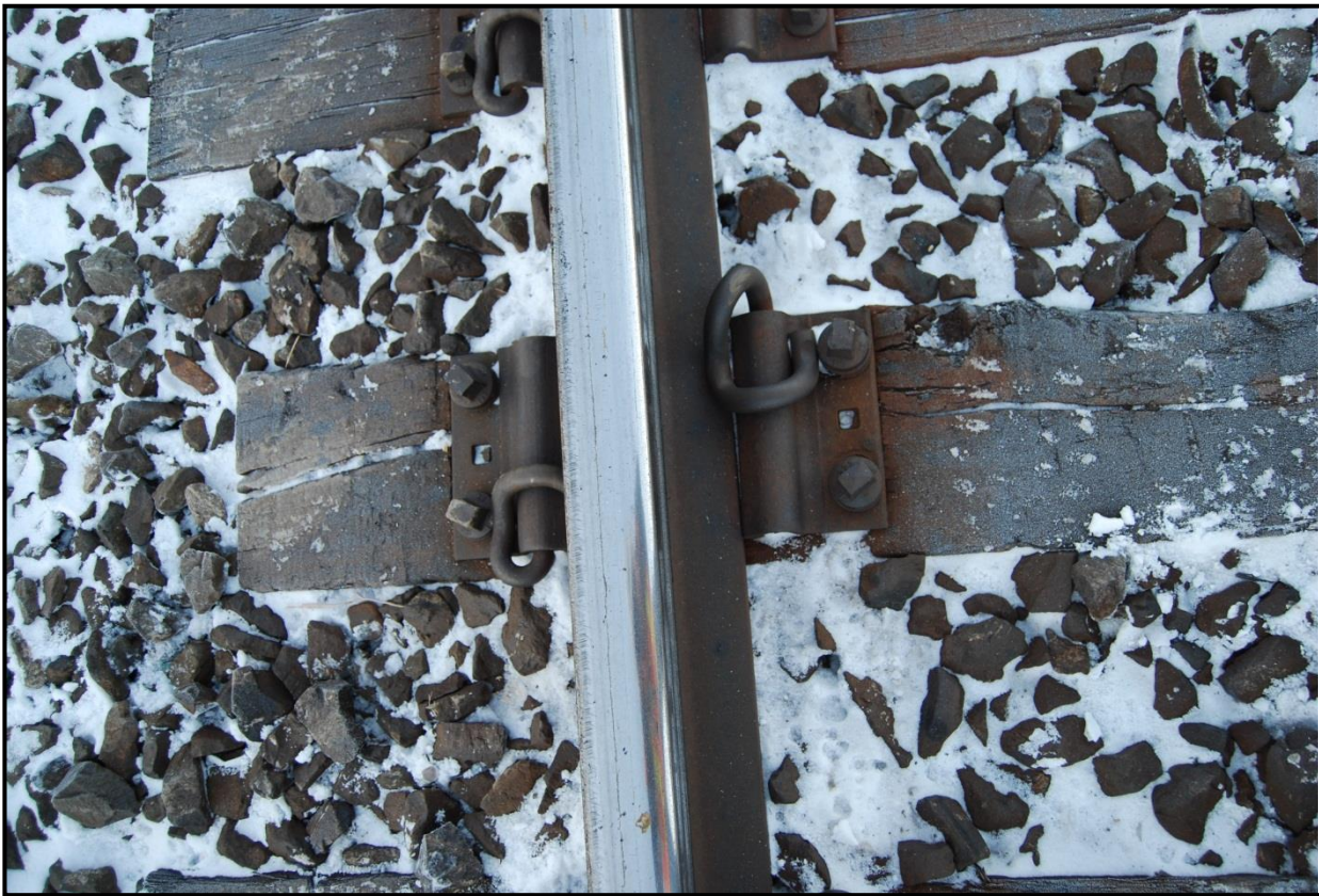
Photo 4. Rolled plate fastener system
