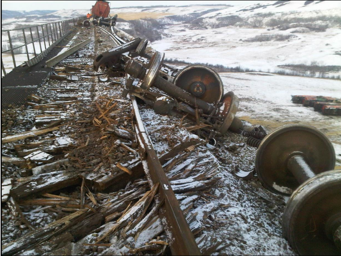
Photo 3. East end of bridge
