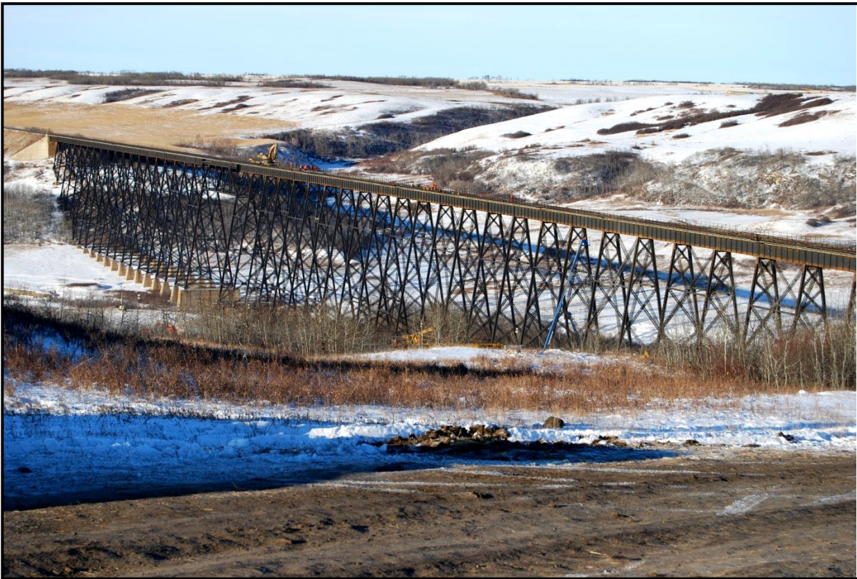
Photo 5. Fabyan Bridge (looking west)
