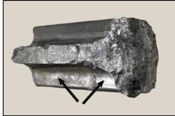
Photo 7. Burnishing under the head of the north switch point rail
