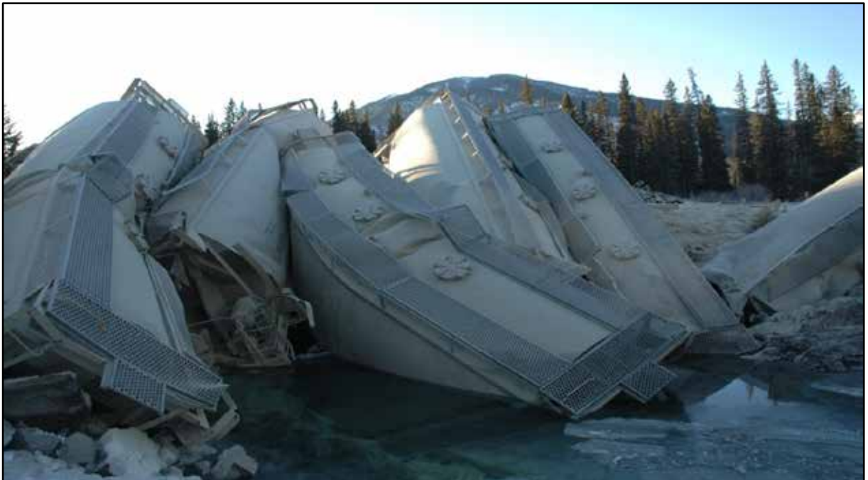
Photo 3. Derailed cars stacked on the bridge
