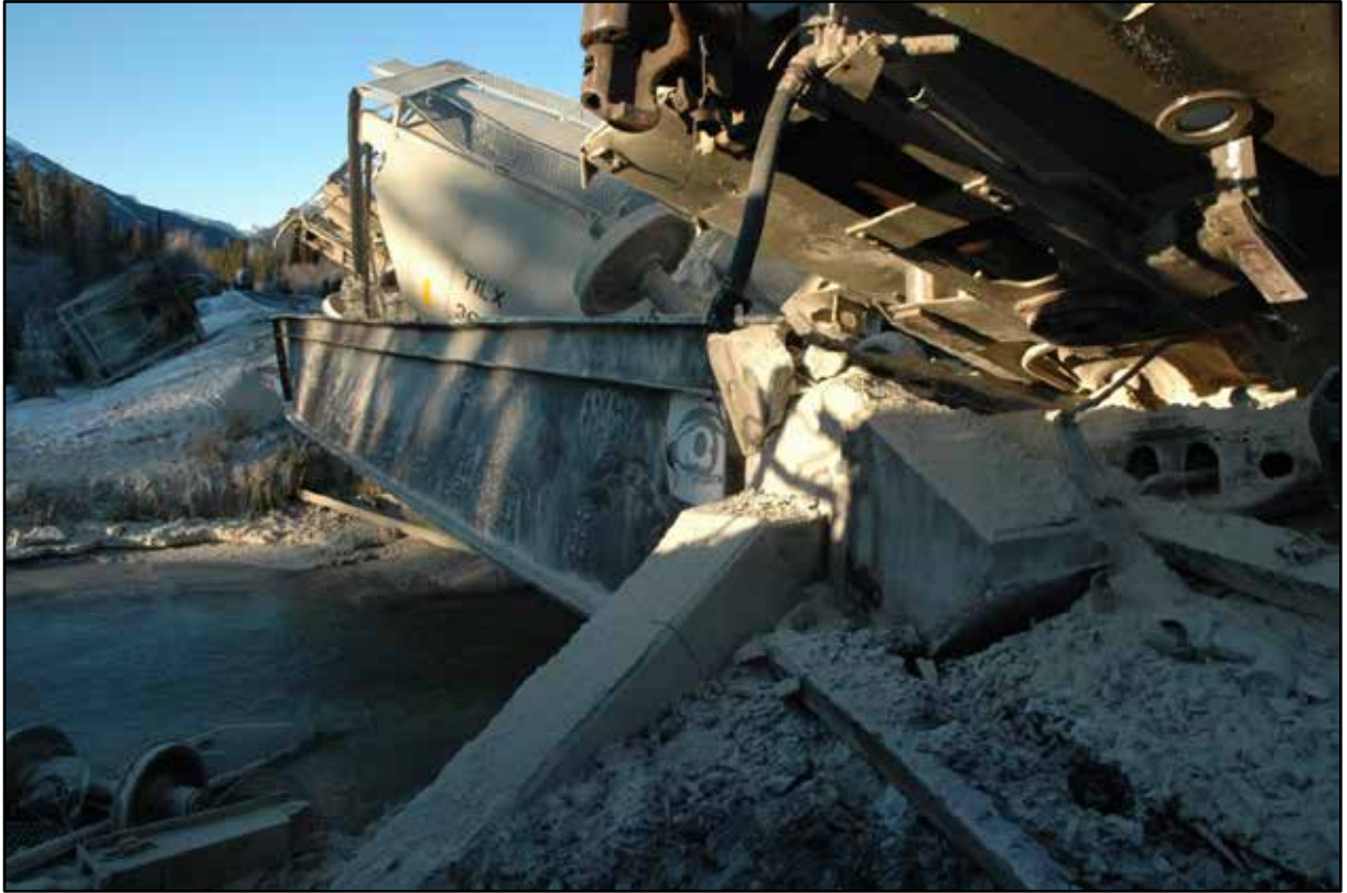
Photo 2. Derailed cars on the bridge
