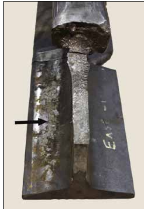
Photo 8. Burnishing on the base of the north switch point rail
