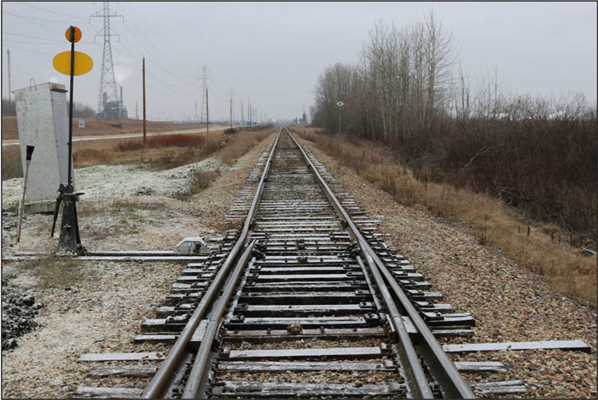
Figure 6. View of the west wye switch in reverse position (looking west)
