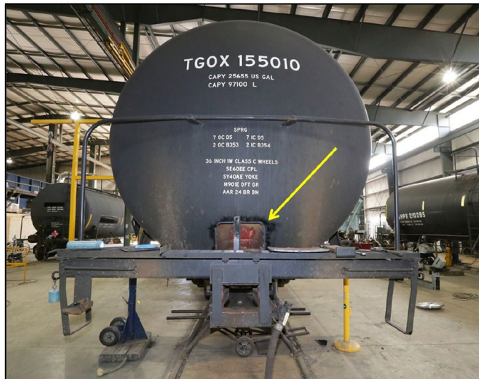
Figure 6. TGOX 155010 prepared for inspection with jacket and insulation removed (arrow)
