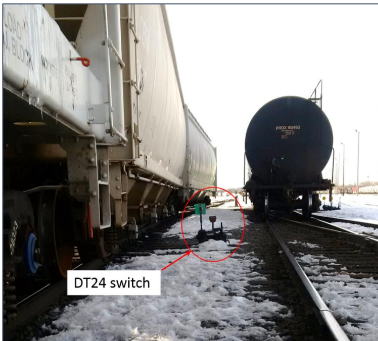
Figure 8. Position of DT24 switch (circled) relative to the adjacent tracks (Source: TSB)
