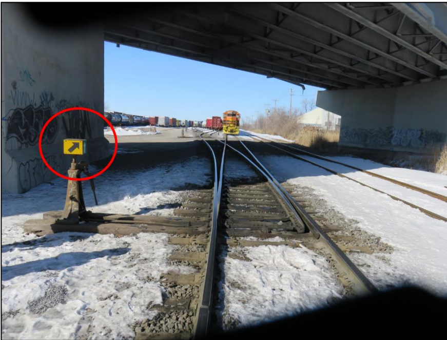
Figure 9. Switch cube direction indicator (Source: TSB)
