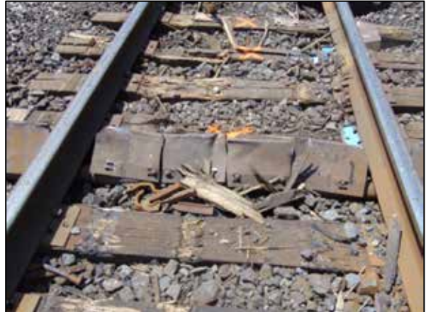
Figure 10. Wheel impact marks on dragging equipment detector deflection paddles (Mile 19.51)
