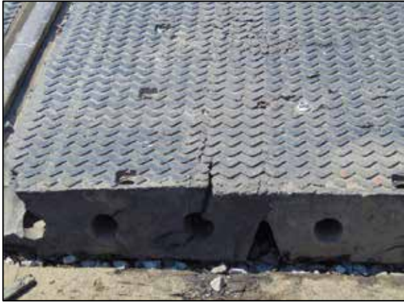
Figure 9. Queen Street crossing rubber surface (Mile 19.50)
