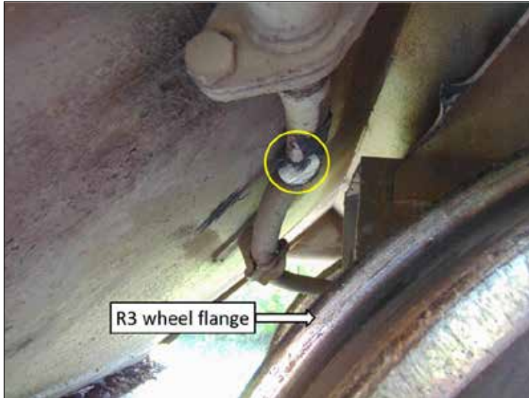
Figure 4. Burn/grind marks on air brake pipe (circled) from contact with the R3 wheel flange (arrow) from car NAHX 35909
