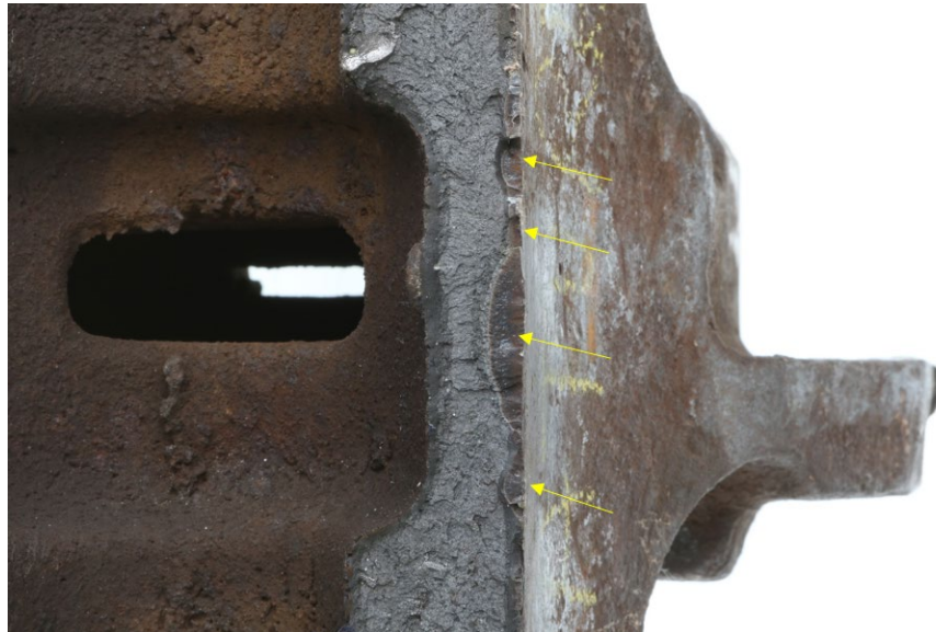
Figure 10. Fatigue cracks (Source: TSB)
